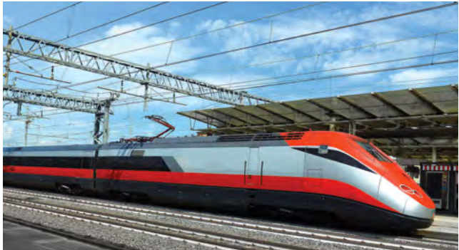
Voltage support systems in railways traction lines
